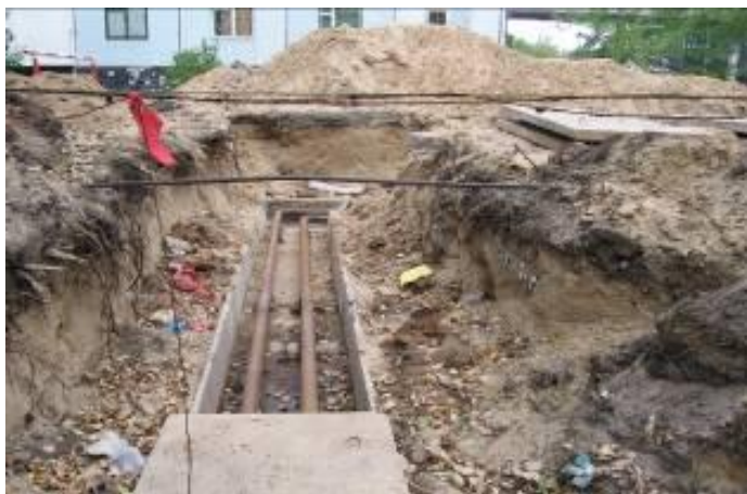
Replacing aged and leaking water pipes
