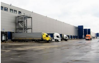
Loading docks – a key component to an industrial park
